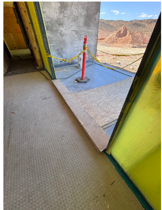
Framed Bridges on top of areas with covered with PRO-TECT Sill tape. Where access is required.
