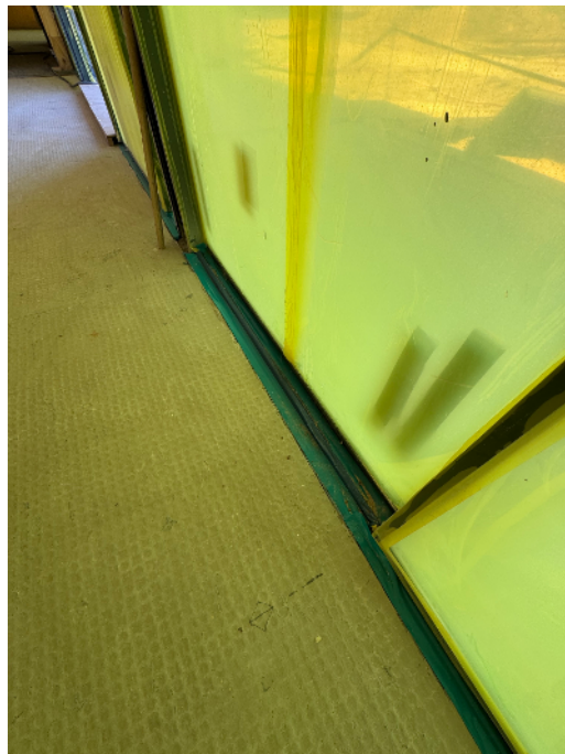
Aluminum Frames protected with PRO-TECT Sill Tape, ceasing debris from entry into wheel tracks
